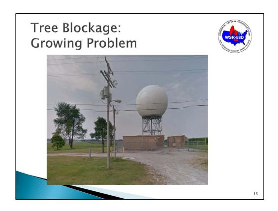
Here is an image from KHPX (Ft. Campbell, KY) from 2013. Note the trees directly next to the radar. It only takes a few trees to cause beam blockage.
